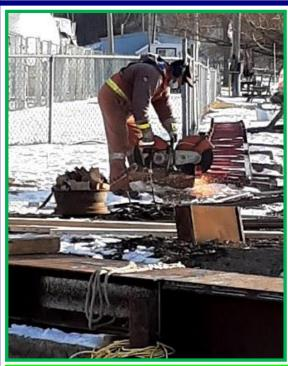
Trimming the girder, drilling and bolting the beams,
