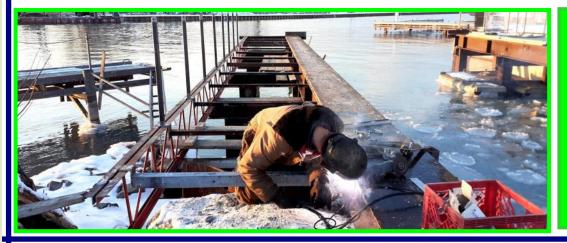
Cross beams installed and welded in next, along with the upright posts for the safety line.
