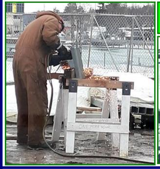
Cutting the rail guide uprights, all stacked and ready to be installed.
